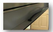
Located approximately 7" down from the top of your mirror, and approximately halfway across on the back side of the mirror, (within the housing) you will find your wire whip (approximately 7" supplied). Here you find a black wire, a white wire, and a green wire. These go to a 115v AC source coming from the bathroom switch, (connect black to black, white to white and green to ground).
